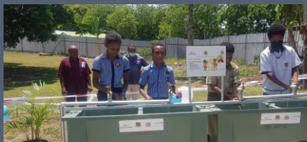
Image: Bore Water supply to Pari Primary School
